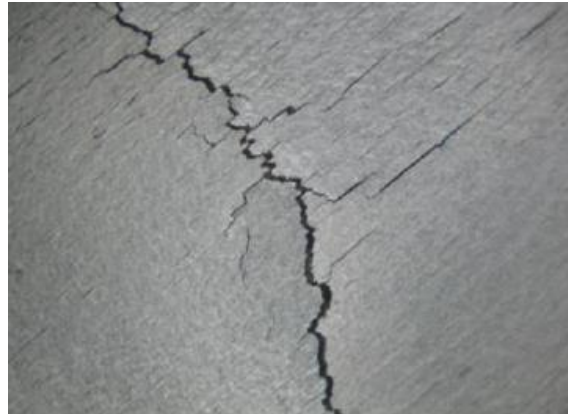
Fig. 3. Cracking in stainless steel.
