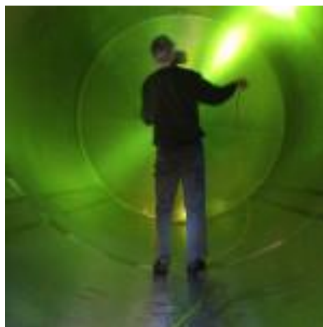
Fig. 8. Inspection with UV-light for cracks and pores in a storage tank.
